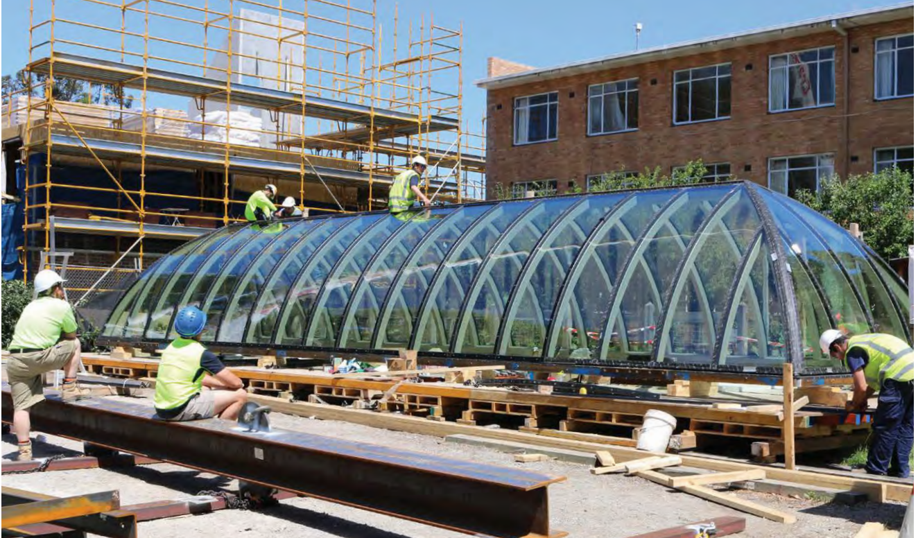
Syme Dining Hall roof construction
